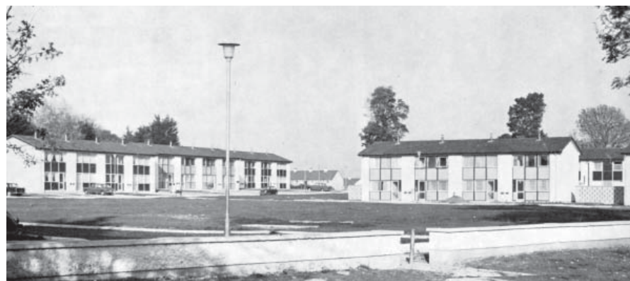
1971 Industrial Housing at Droichead Nua
