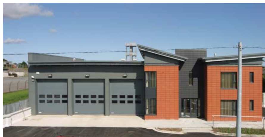
Wexford Fire Station
